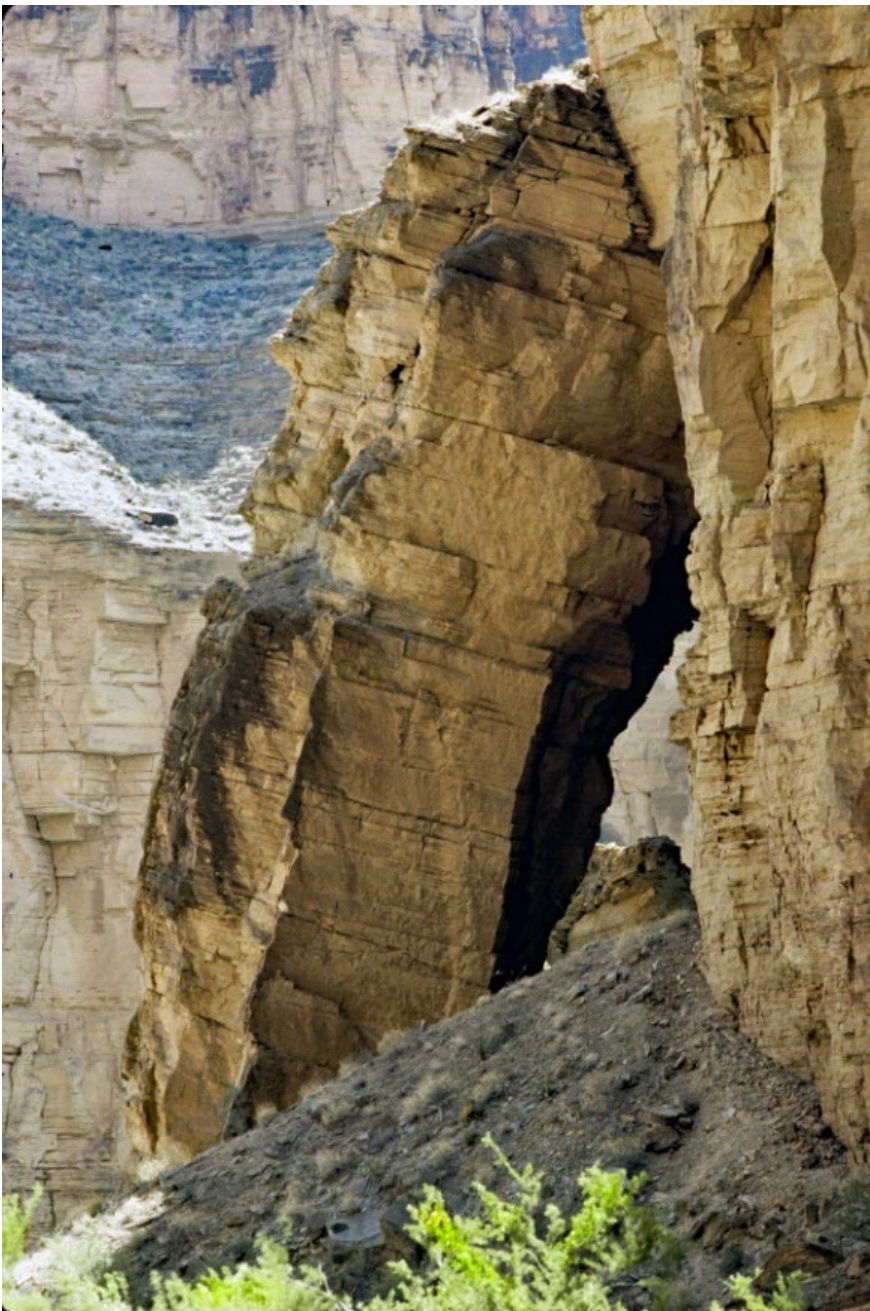
Fig. 21.2. "The Leaning Pillar of Fern Glen" viewed southwest from the mouth of that famous slot canyon. A huge pillar of Muav Limestone defined by more than four fracture surfaces has dropped off the wall and "heeled out" over the Bright Angel Shale. This is a stunning example of how erosion in the Grand Canyon initiates not grain-by-grain but rather block-by-block.
