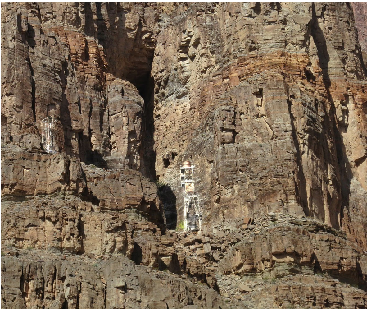
Fig. 22.11. Abandoned terminal for cable that extended across the river and 3,000' up to the south rim. Gondolas filled with guano from Bat Cave were to be hefted up to trucks that would carry it to Kingman. After 1,000 lbs were delivered, all was abandoned. An Airforce jet severed the cable in 1960.
