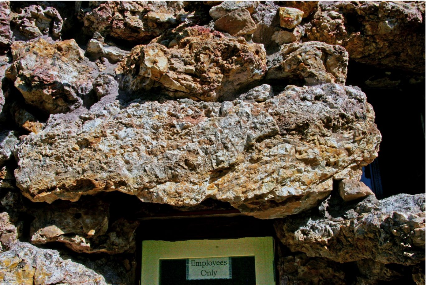
Fig. 3.10. Close up of chert/agate rubble at the base of the Watchtower. These large building blocks were quarried out of the top surface of the Kaibab Limestone at this location. The fresh surfaces allow convenient examination of the internal nature of a paleokarst chert residuum.
