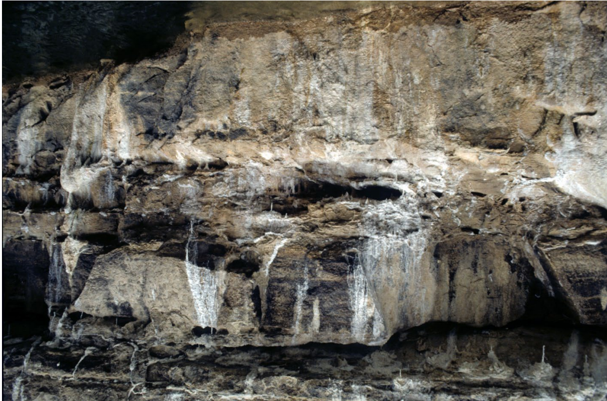
Fig. 12.16. Where the rock face can be seen along the salt walls, highly weathered sandstone is apparent. The rock is completely rotted, with elongated zones and even thin beds where the sand grains washed out. Such intense weathering of sandstones is rare. The elongated opening in the direct center is about 3 inches high.
