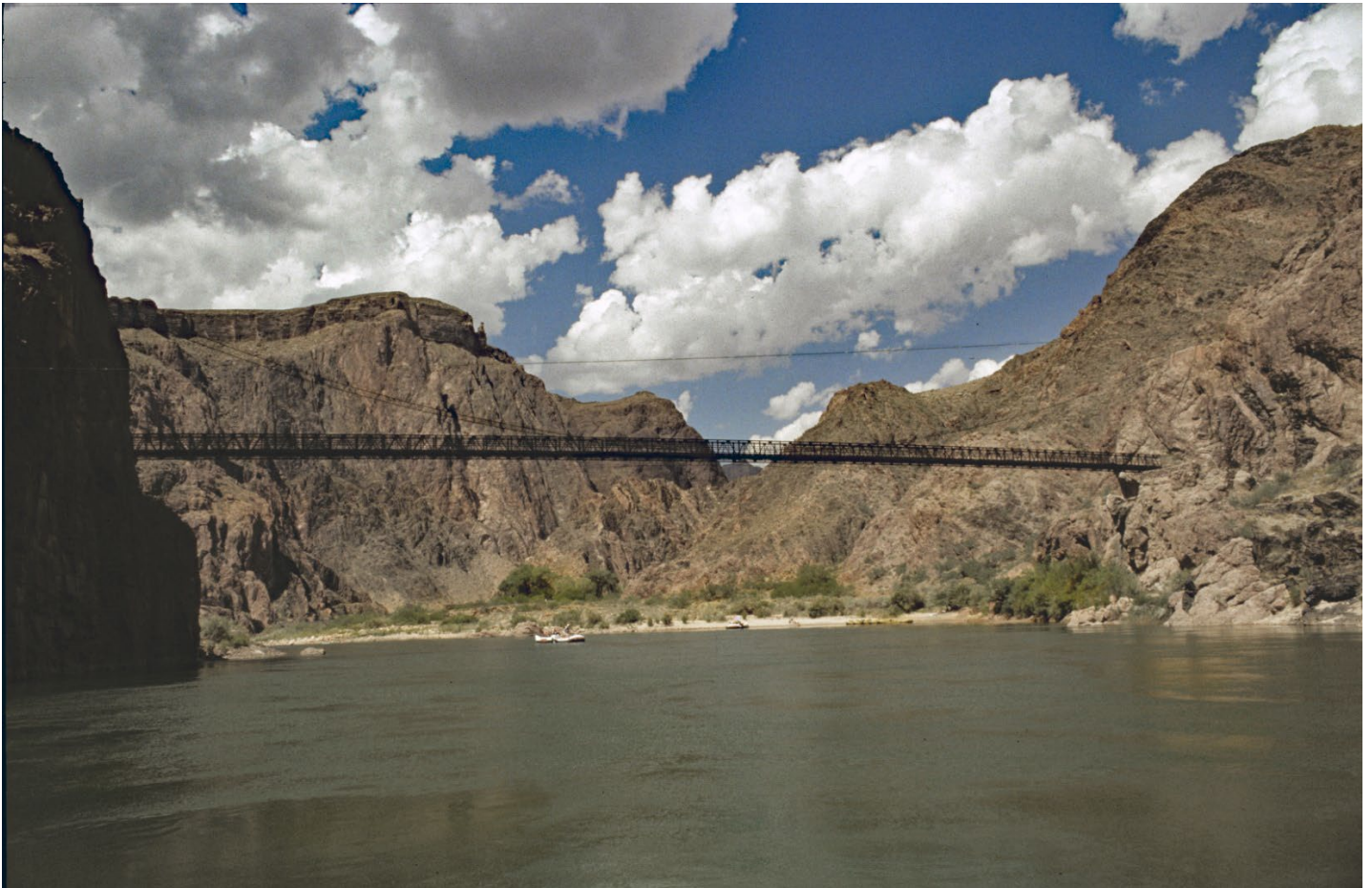
Fig. 16.17. Suspension bridge connecting the South Kaibab Trail to a short trail to Phantom Ranch. Another suspension bridge about one mile downstream connects Phantom Ranch to the Bright Angel Trail going up to the South Rim. Note the thin cable running above the bridge from which a small trolley used to carry operators out to the center of the channel to measure flow rates.
