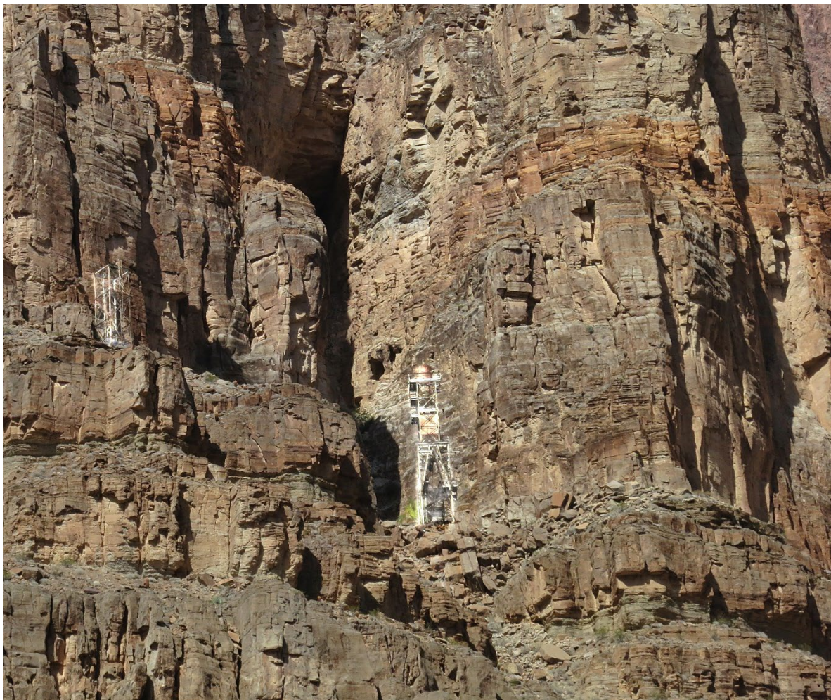
Fig. 22.11. Abandoned terminal for cable that extended across the river and 3,000' up to the south rim. Gondolas filled with guano from Bat Cave were to be hefted up to trucks that would carry it to Kingman. After 1,000 lbs were delivered, all was abandoned. An Airforce jet severed the cable in 1960.
